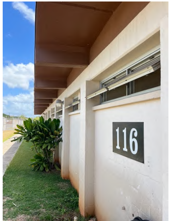
Bathroom window caulking tested; no asbestos detected
