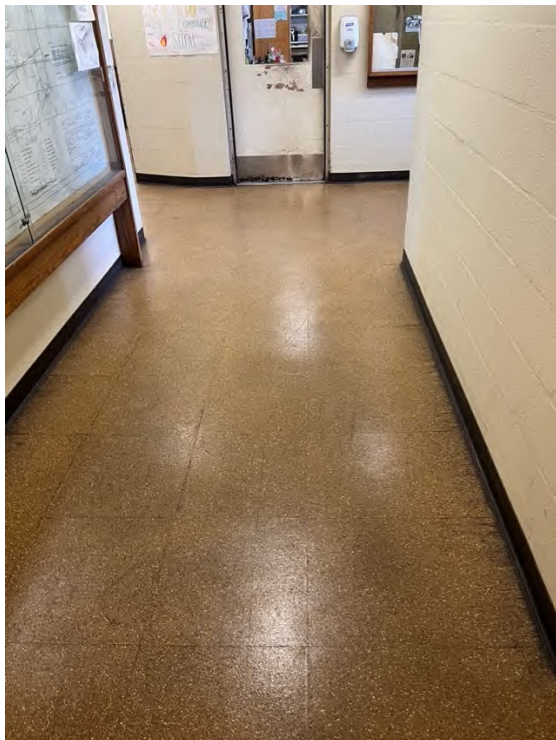
Brown speckled VFT/Mastic, and brown cove base/mastic; no asbestos detected
